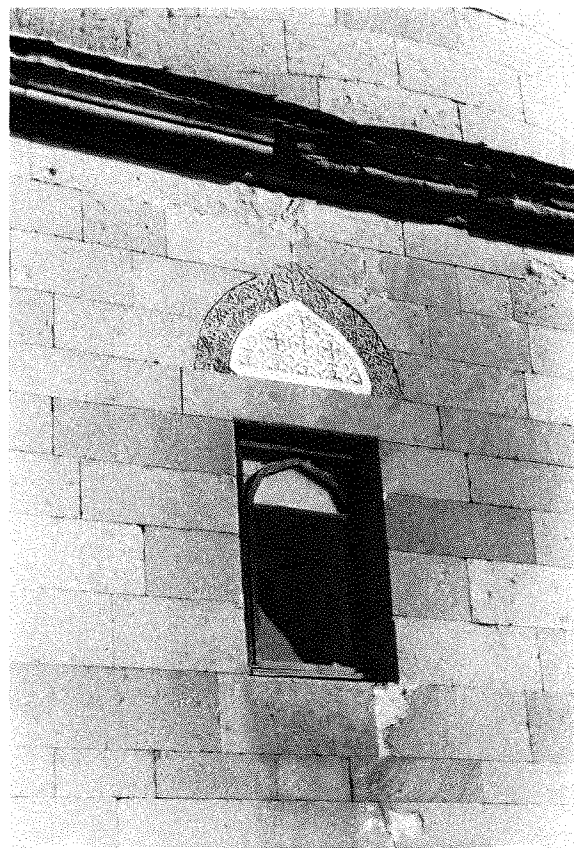
6 — Kumanovo, Mosque of Tatar Sinan Bey, detail of masonry and decoration.
